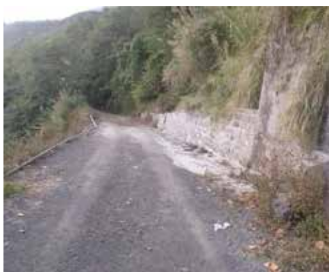
Construction of the retention wall in Porba station to prevent landslide
