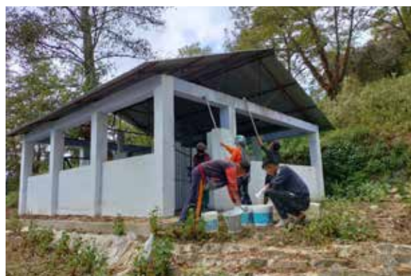
Completed renovation and painting of the Mithun Farm at Porba Station
