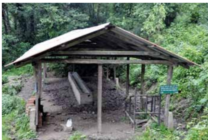
Figure 13: Modified Travis installed in the farmer's field
